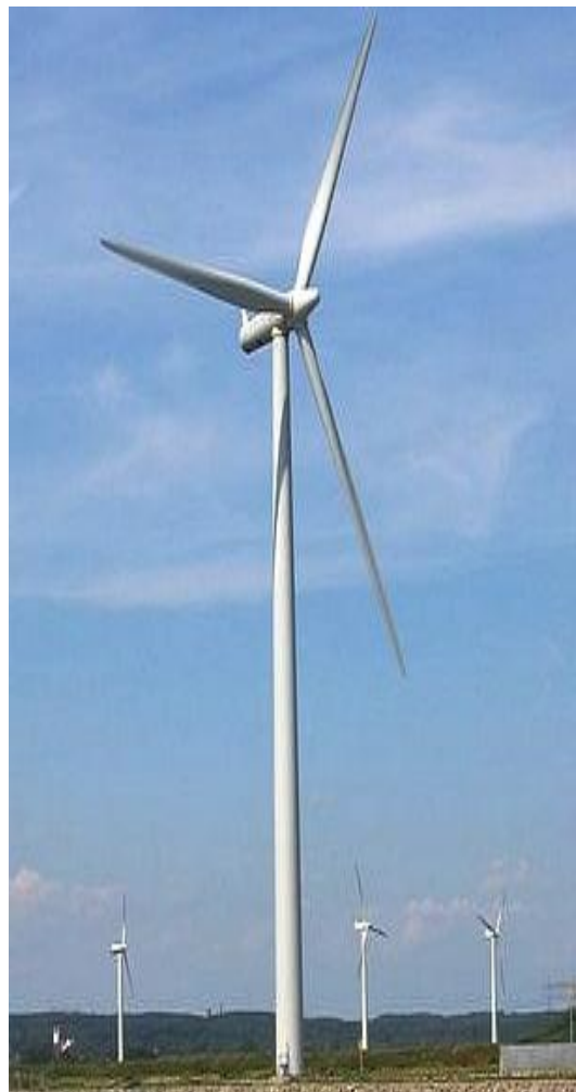
Proposed turbines at Anderby (127 metres)
